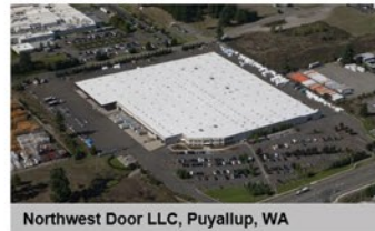
Northwest Door LLC, Puyallup, WA
